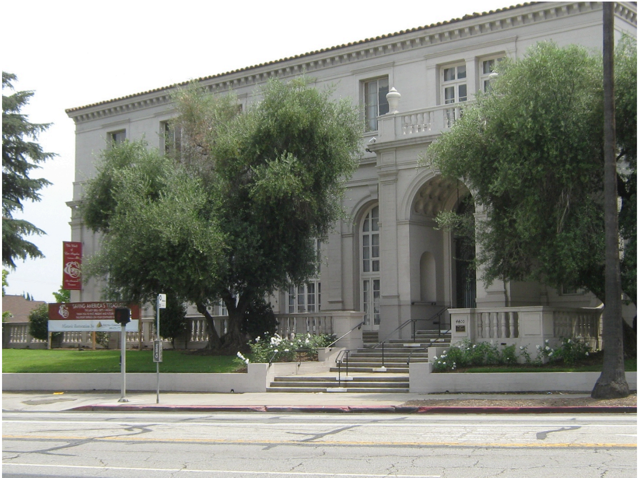
The Ebell of Los Angeles entrance at Wilshire Boulevard. Photo by Libby Simon. July 20, 2013.
