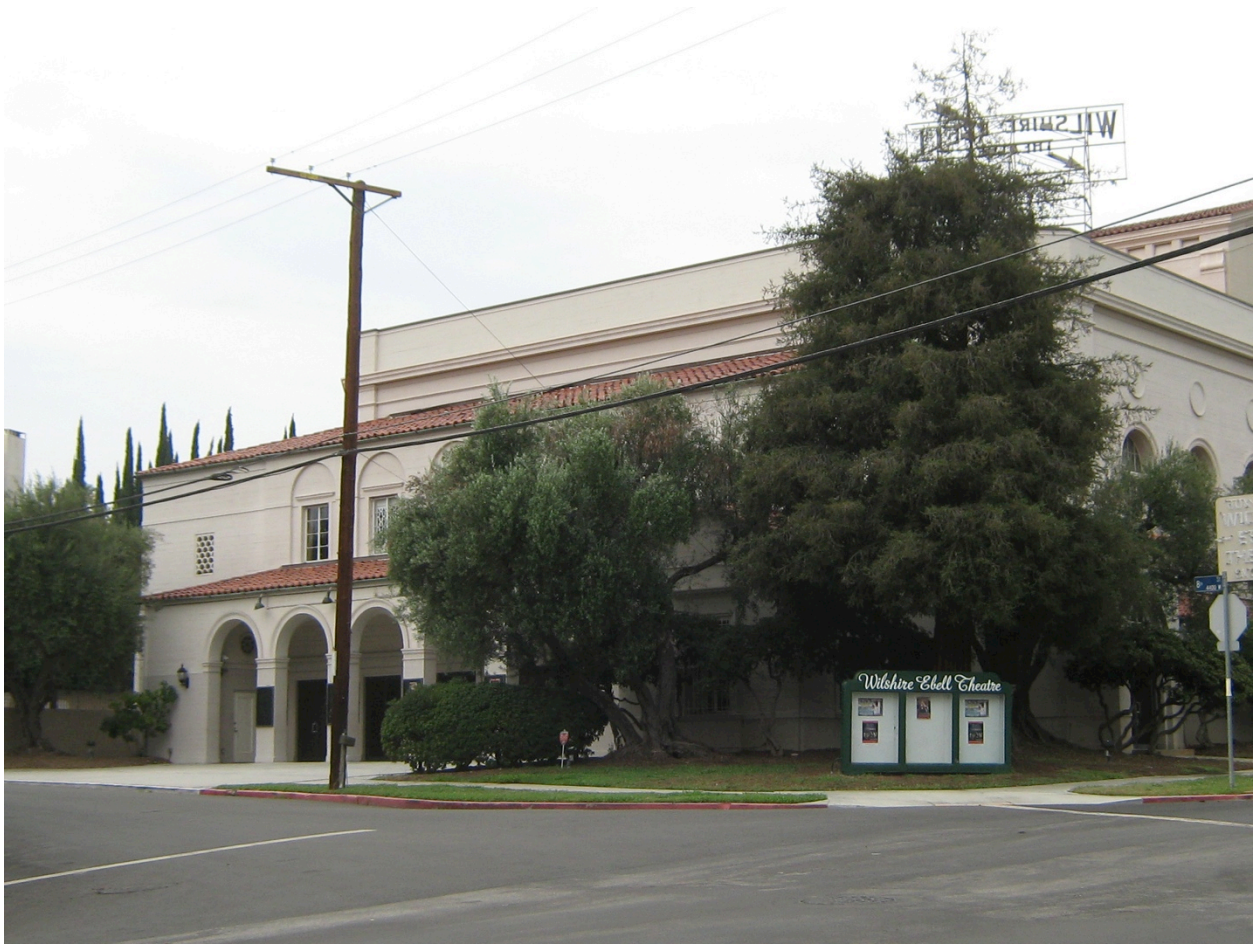
The Ebell of Los Angeles, south elevation, The Wilshire Ebell Theatre entrance. Photo by Libby Simon. July 11, 2013.
